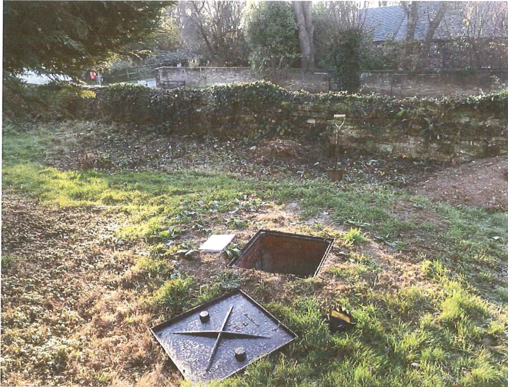
Location of soakaway within church yard.
